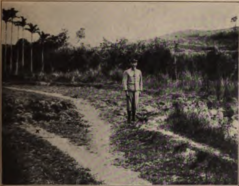
A. An earthquake fault opened in Formosa in 1906, with vertical and lateral displacements combined (after Omori).
